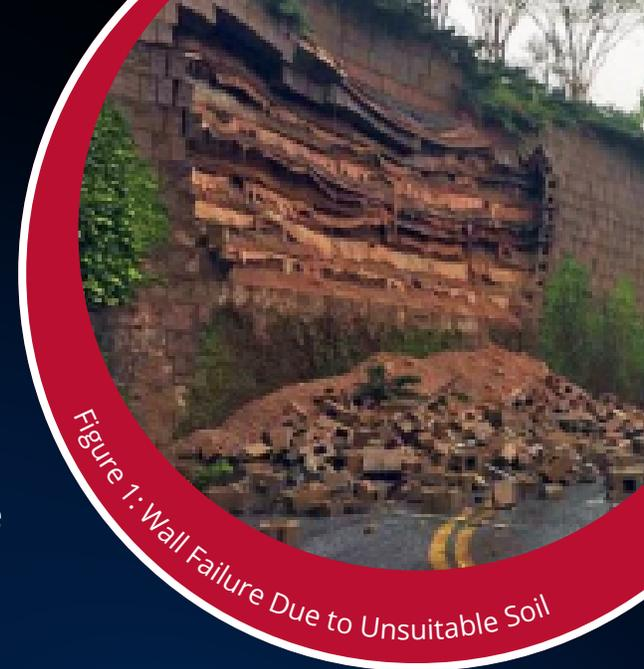
Figure 1: Wall Failure Due to Unsuitable Soil
