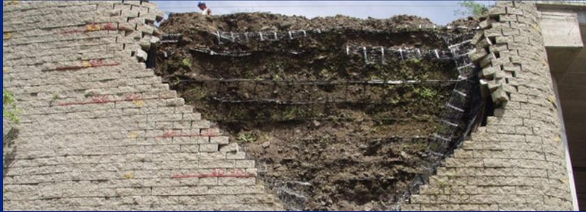
*Figure 6: Wall Failure Due to Improper Quality Control*
