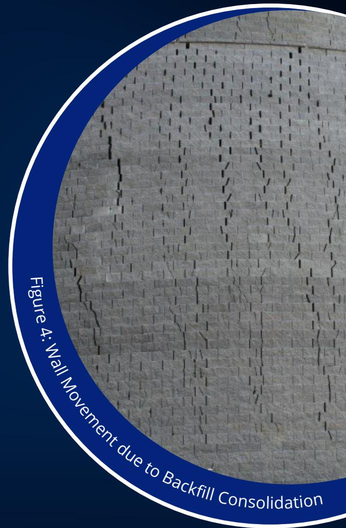
Figure 4: Wall Movement due to Backfill Consolidation
