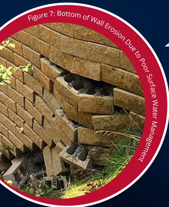
Figure 7: Bottom of Wall Erosion Due to Poor Surface Water Management
