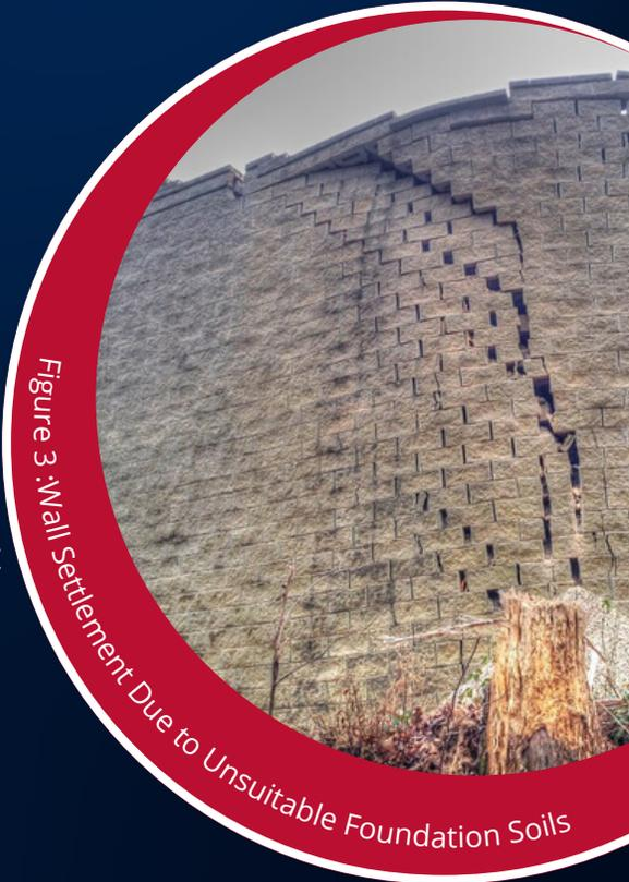
*Figure 3 : Wall Settlement Due to Unsuitable Foundation Soils*
